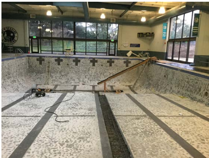
(concrete backfill over new pipe inside the pool)
