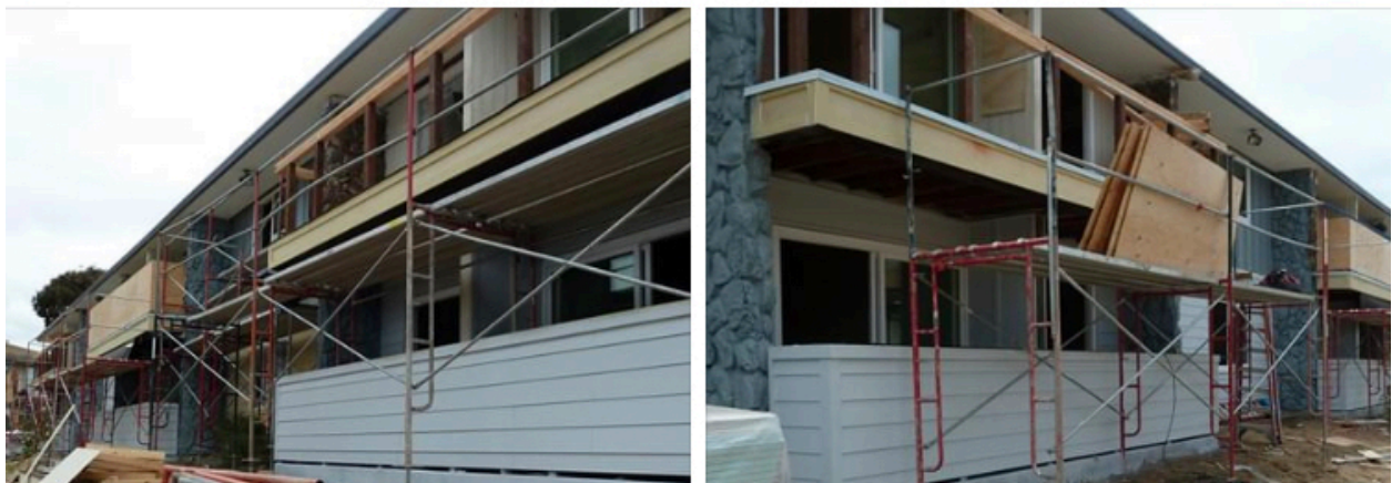
Del Monte Manor Renovation Facebook Post
