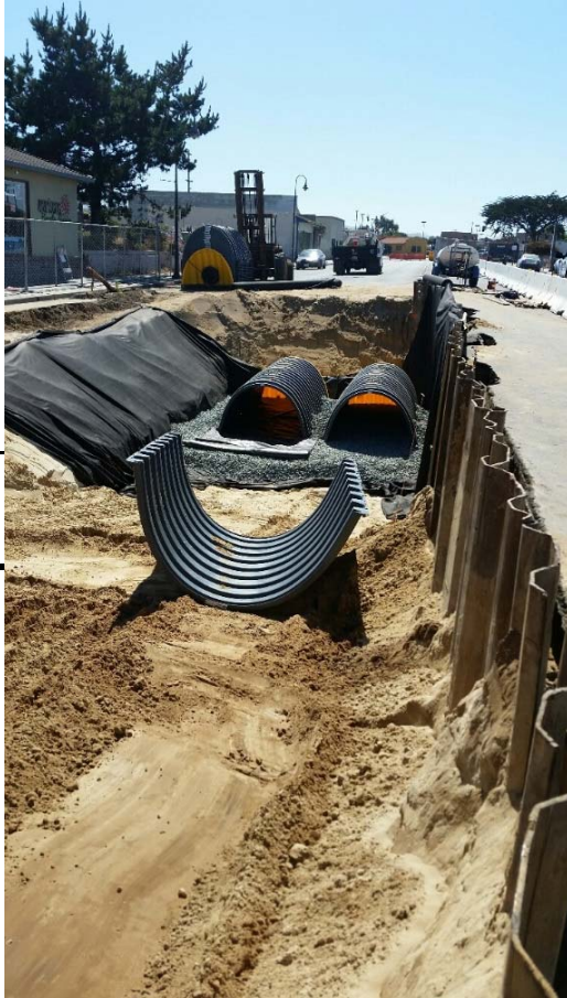
Infiltrator segment placement, Infiltrator #1
