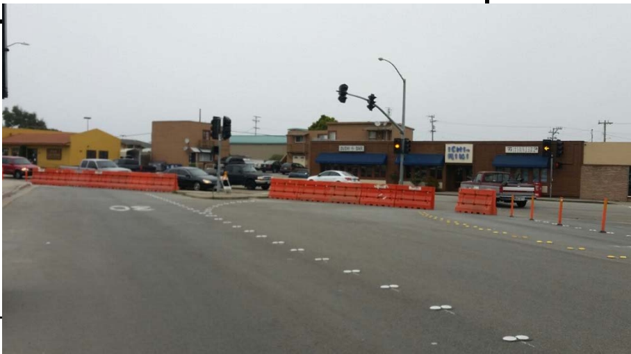
West Broadway closure at Del Monte Ave
