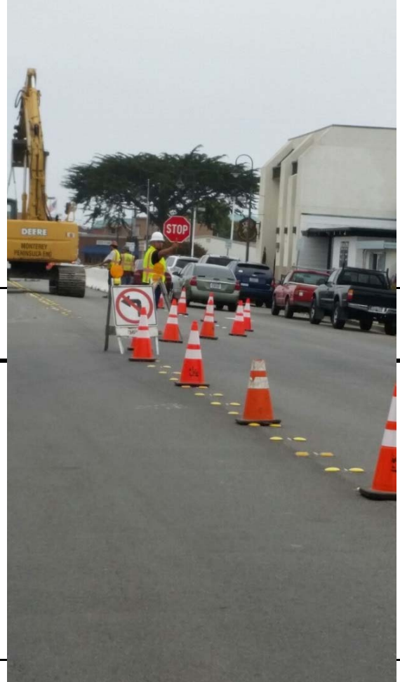
Traffic control for K rail placement
