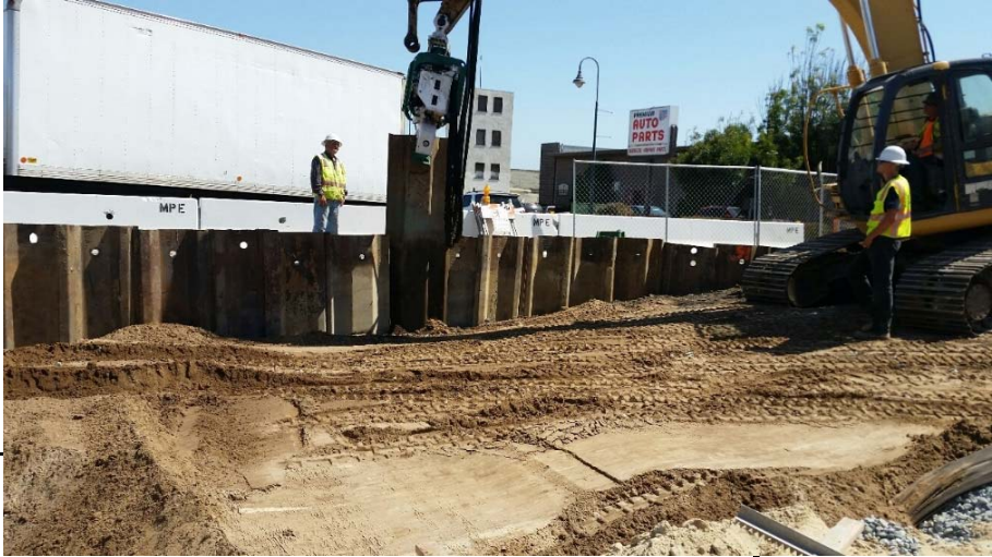
Start of sheet pile removal, Infiltrator #1
