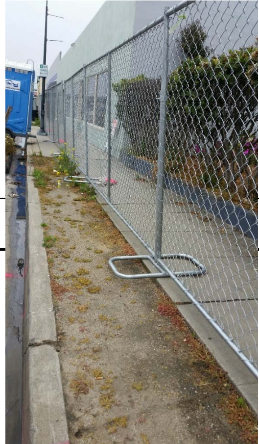
Temporary pedestrian fencing
