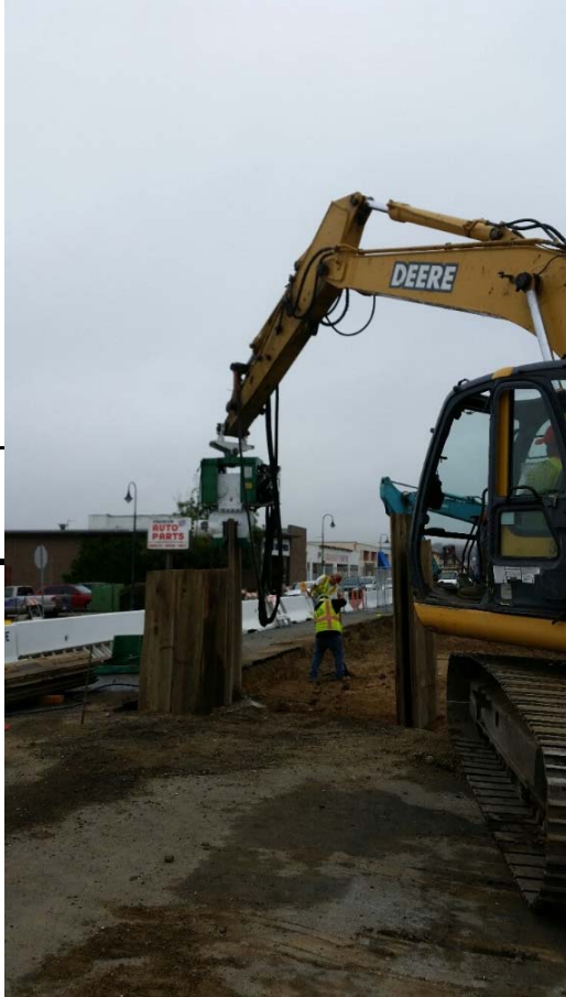
Sheet pile driving, Infiltrator #1
