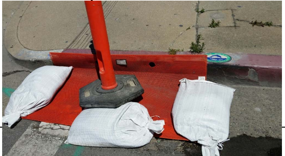
Drainage inlet protection
