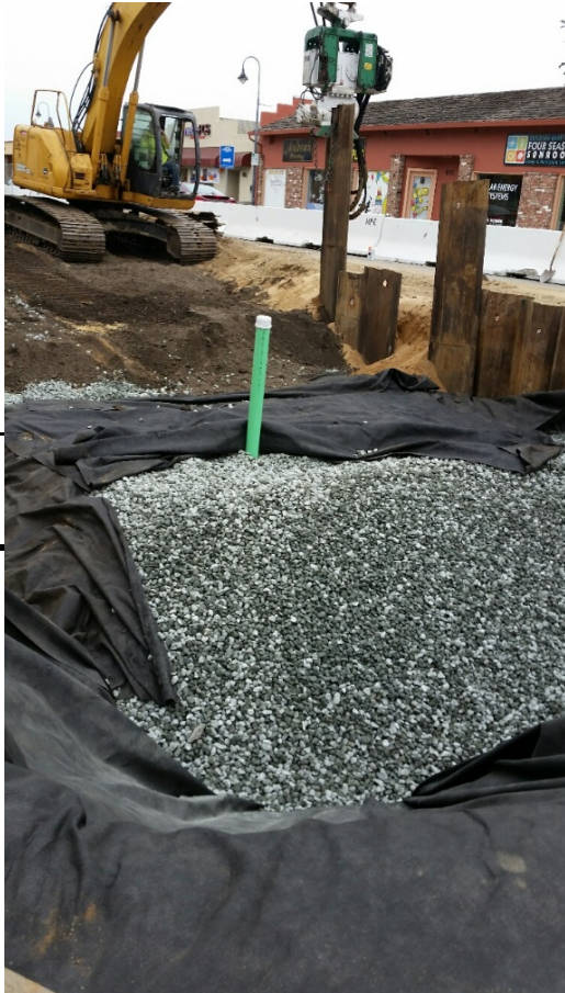
Final rock backfill, Infiltrator 4 closed end; sheet pile removal
