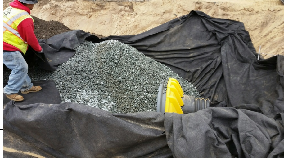
Temporary backfill of inflow end of Infiltrator #4
