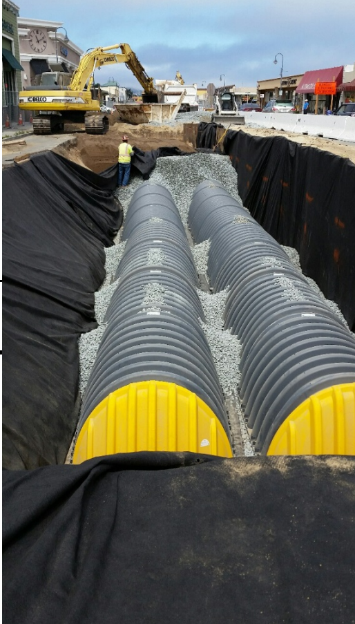
Backfill, Infiltrator #4
