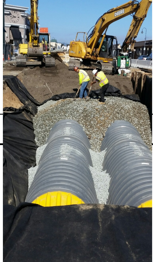
Backfill, Infiltrator #4
