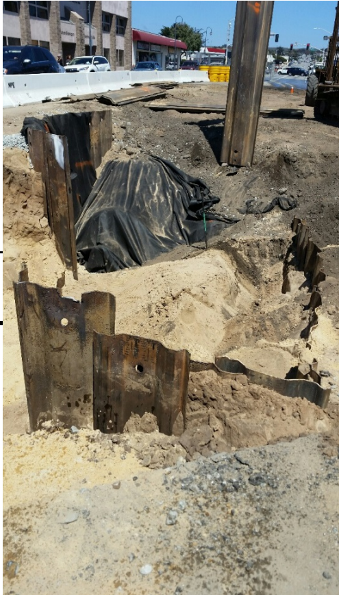
Sheet pile installation, HDS and weir excavation west of Infiltrator #4
