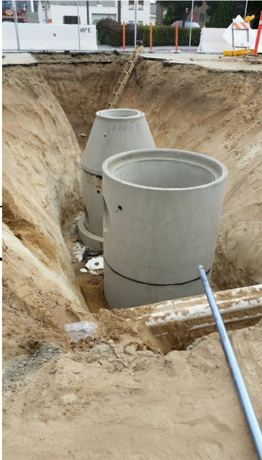
Drainage Structures 1E and 1T
