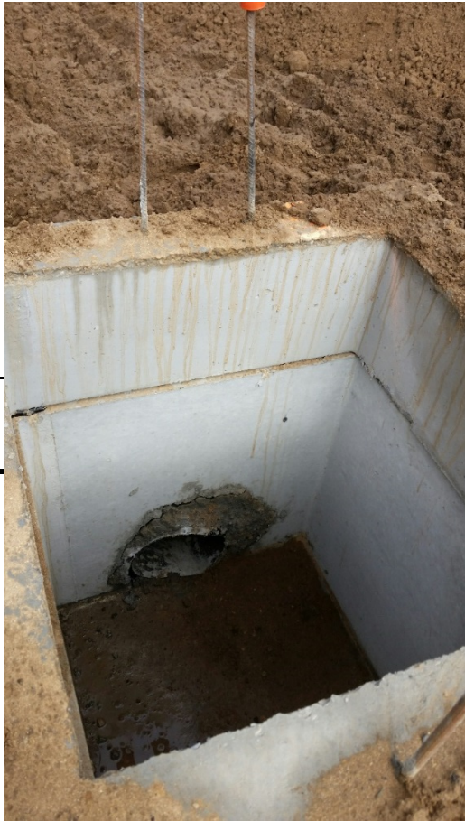
Drainage Structure 1U, backfilled with pipe installed
