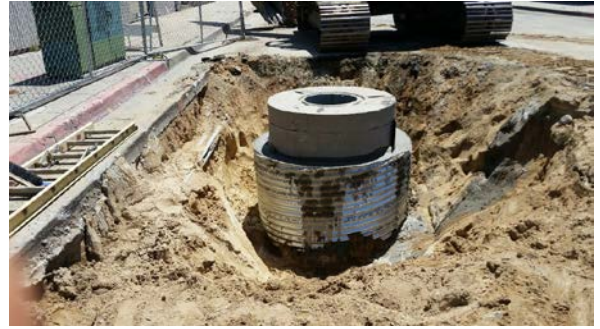
CMP forms for slurry backfill/sealing, DS 1P
