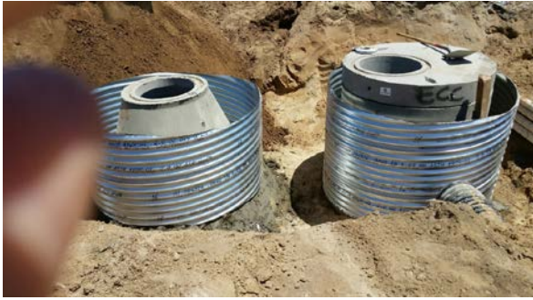
CMP forms for slurry backfill/sealing, DS 1E and 1T
