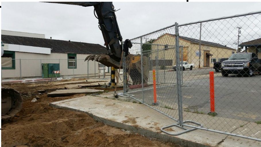
Sidewalk and AC demolition, Hillsdale St
