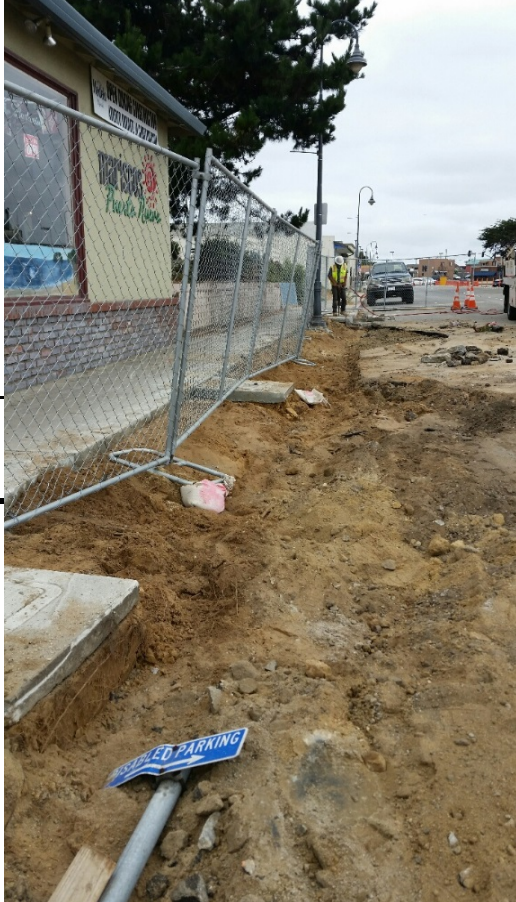
Sidewalk demolition west of Hillsdale St
