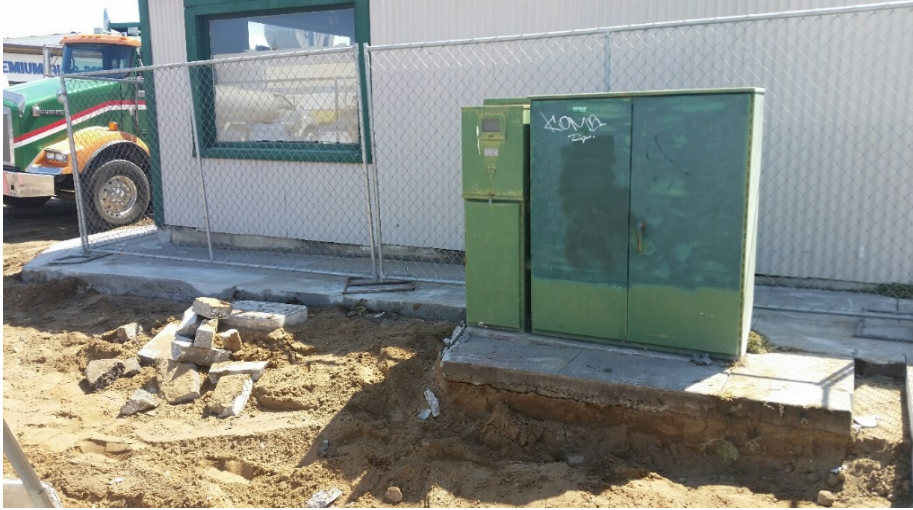
Sidewalk and Curb and Gutter demolition, Hillsdale St west side
