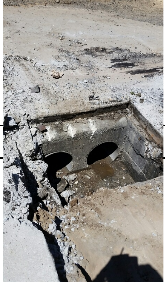
Drainage Inlet removed, southeast corner of Alhambra St
