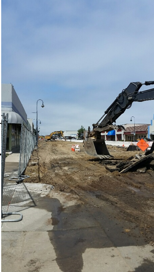
Excavation for Drainage Structure 2, Alhambra St
