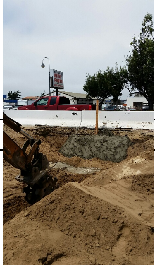
Excavation for DS 1a, stabilized at the existing roadway/k-rail
