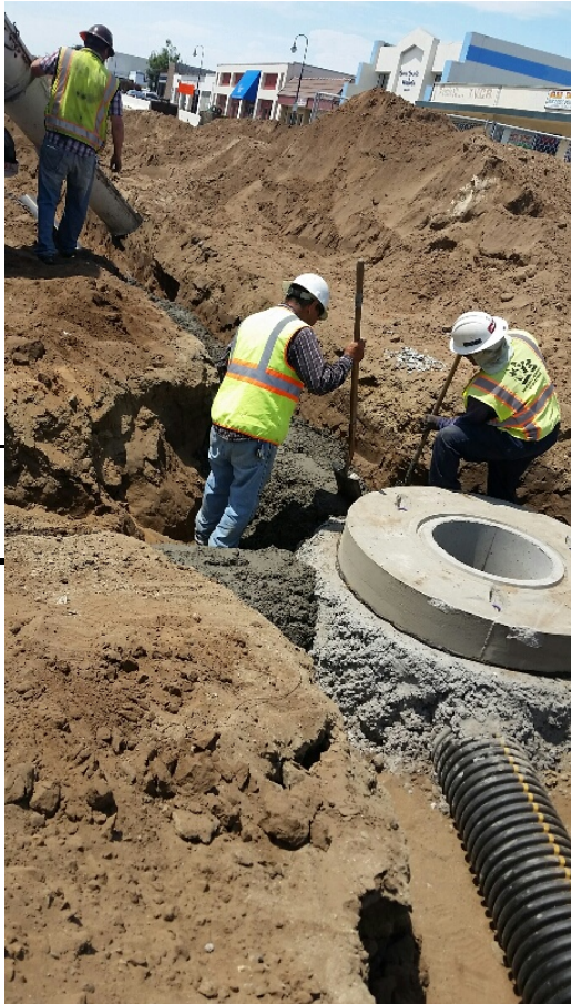
Concrete backfill at pipes connecting to DS 4c
