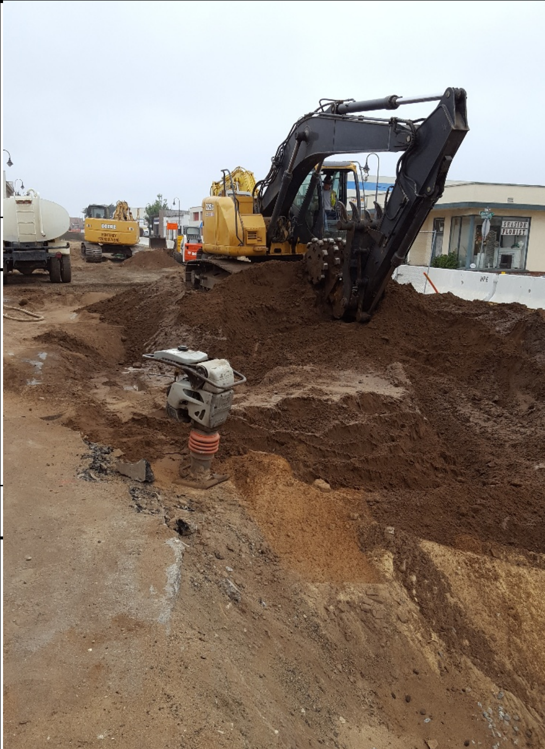
Backfill on Main Stree
