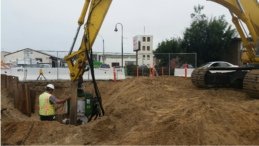
Driving piles, west of Infiltrator #1
