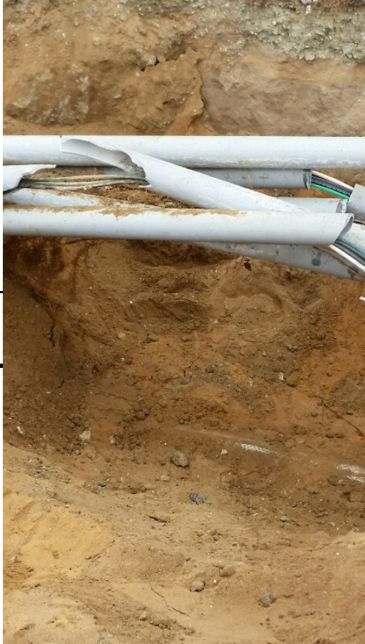
Conflict with electrical and irrigation conduit, DS 6d
