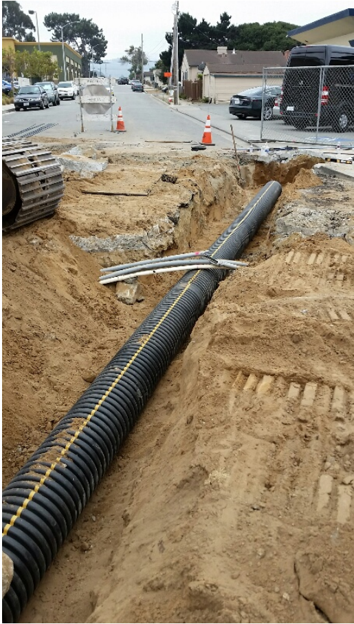
Drainage pipe 6 d, beneath electrical and irrigation conduit
