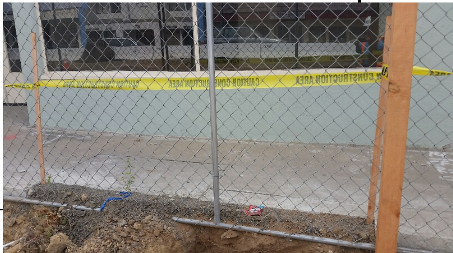
Existing electrical conduit removal, between Hillsdale and Alhambra Streets
