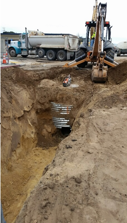
Excavating for Drainage Structure 6d, 12" HDPE pipe
