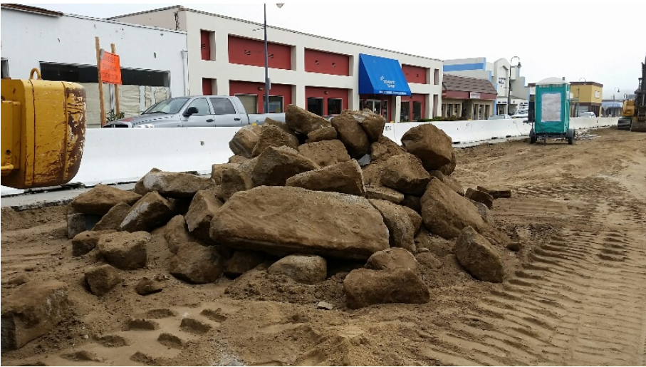
Cement slurry removed and stockpiled
