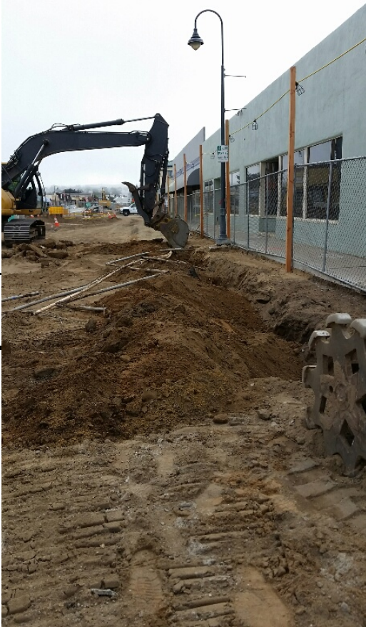
Removal of elect/irrig conduit and cement slurry east of Hillsdale St
