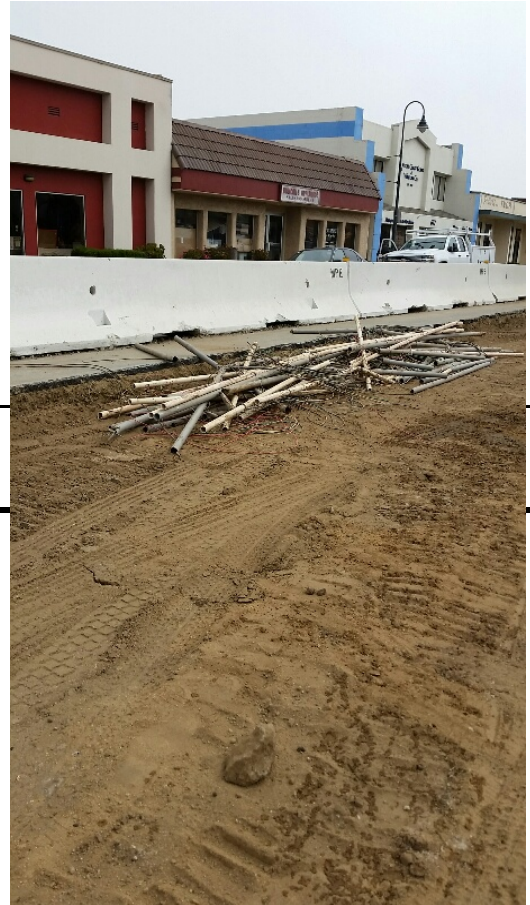
Electrical and irrigation conduit removed and stockpiled
