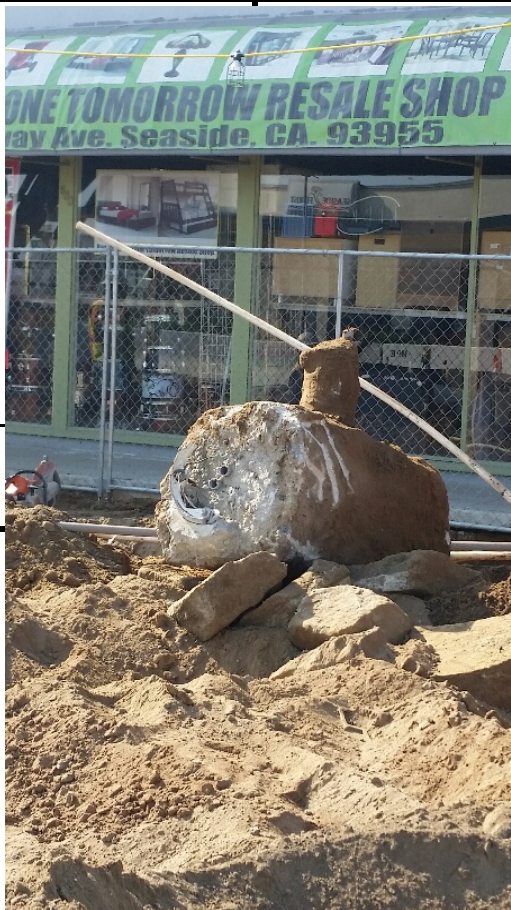
Streetlight foundation removed
