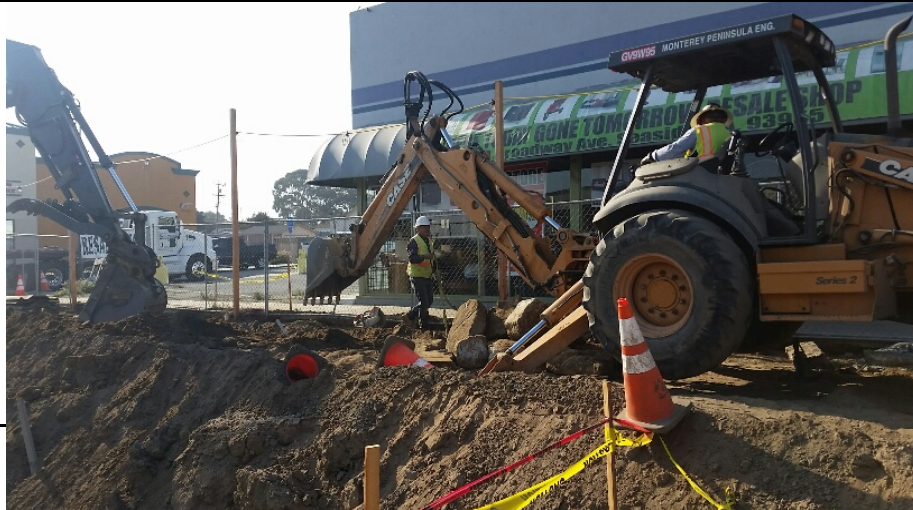
Concrete slurry removal near Alhambra St.
