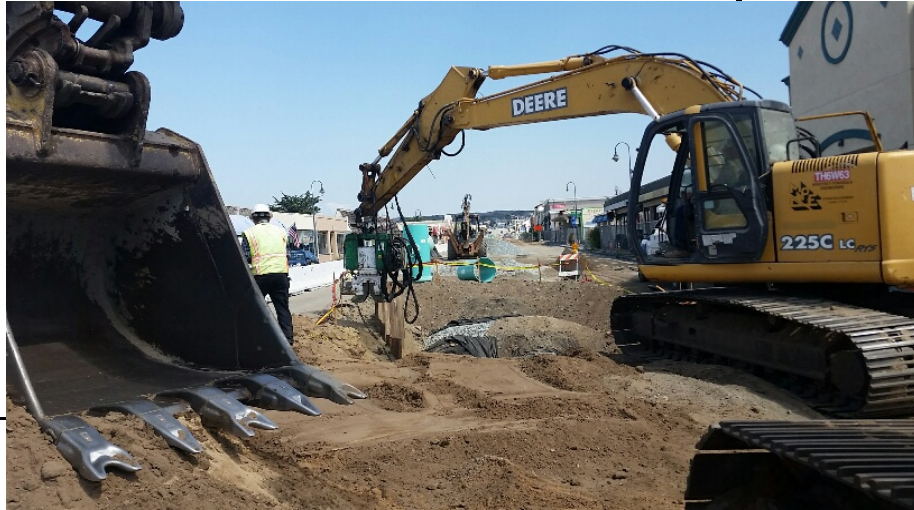
Sheetpile installation Infiltrator #2
