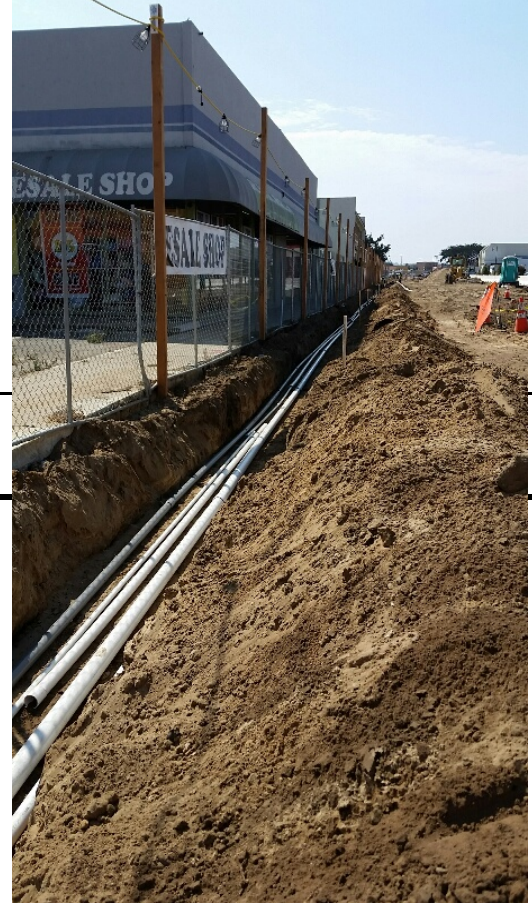
Irrigation trench with electrical and water conduit, west of Alhambra St
