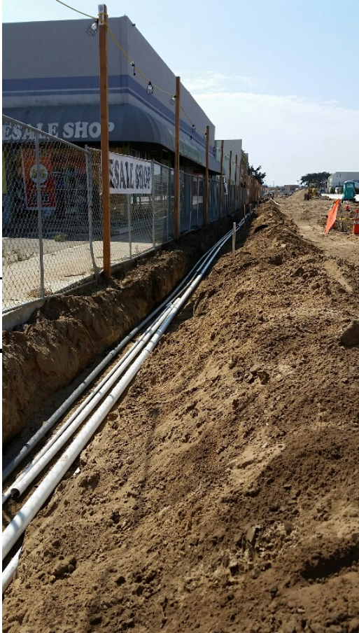
Irrigation trench with irrigation and electrical conduit, west of Alhambra St
