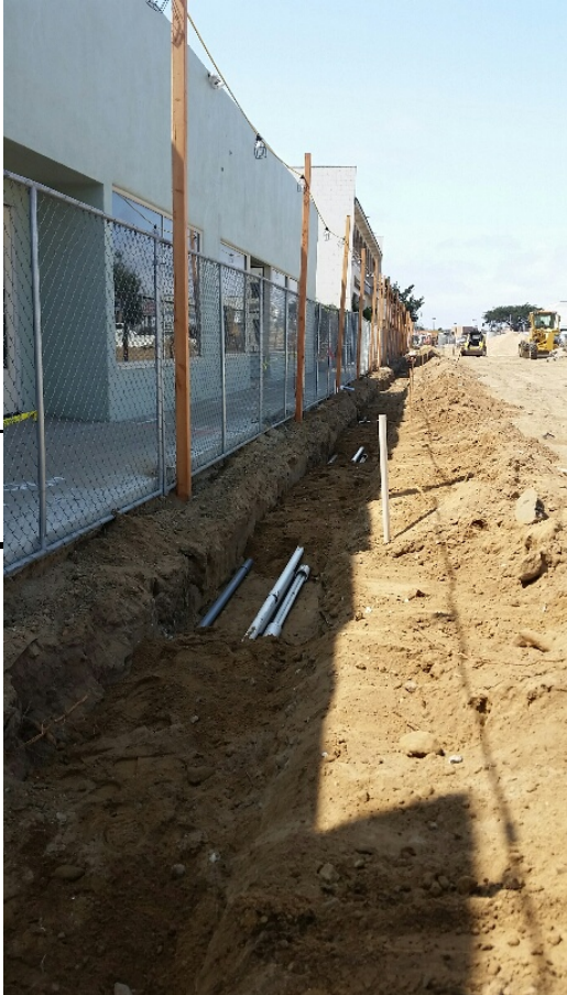
Irrigation conduits, looking west from Alhambra St
