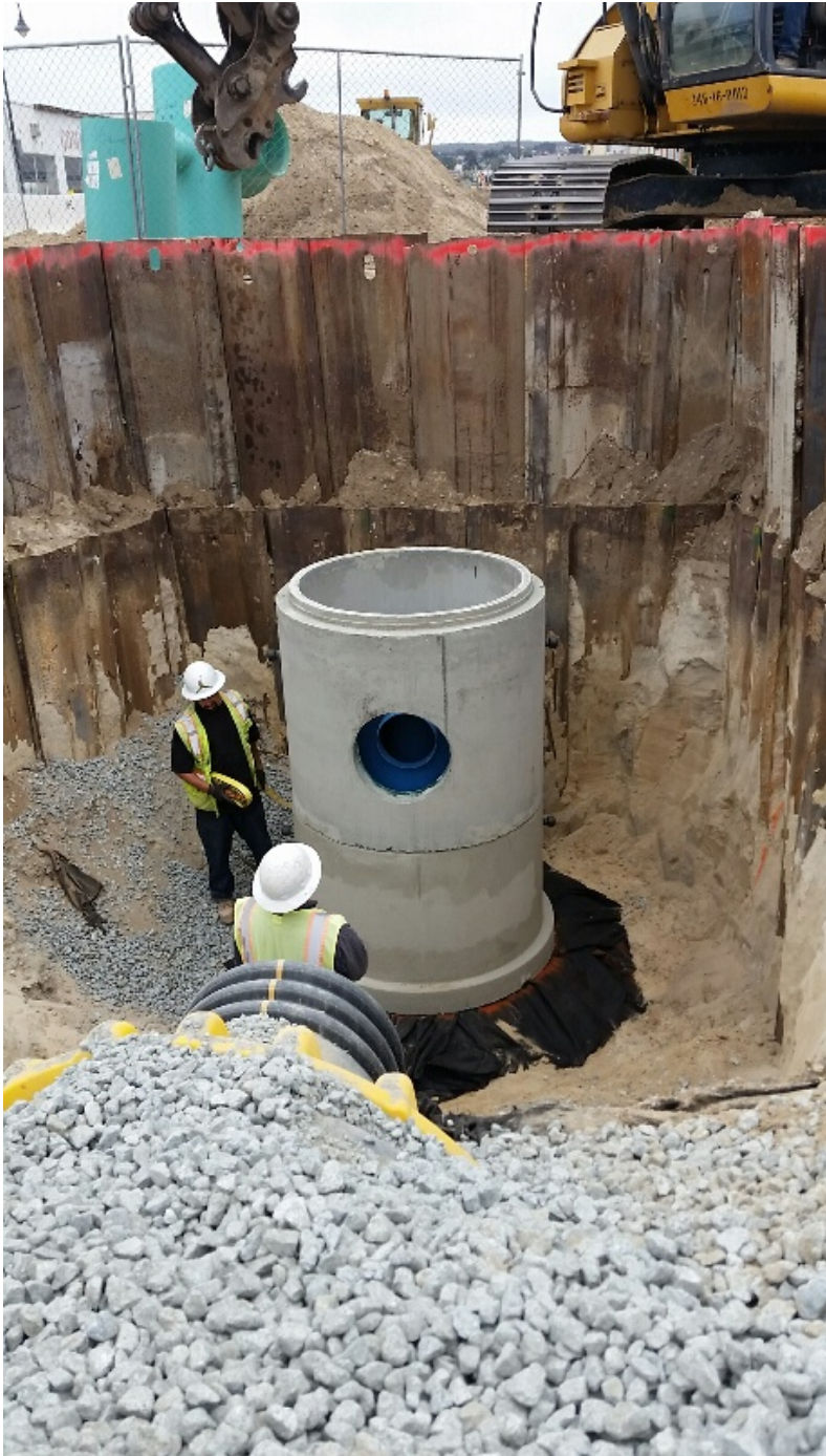
Hydrodynamic Separator #1 installation
