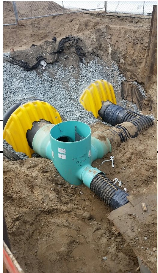
Pipe connections between HDS #1, weir and infiltrator partial backfill only
