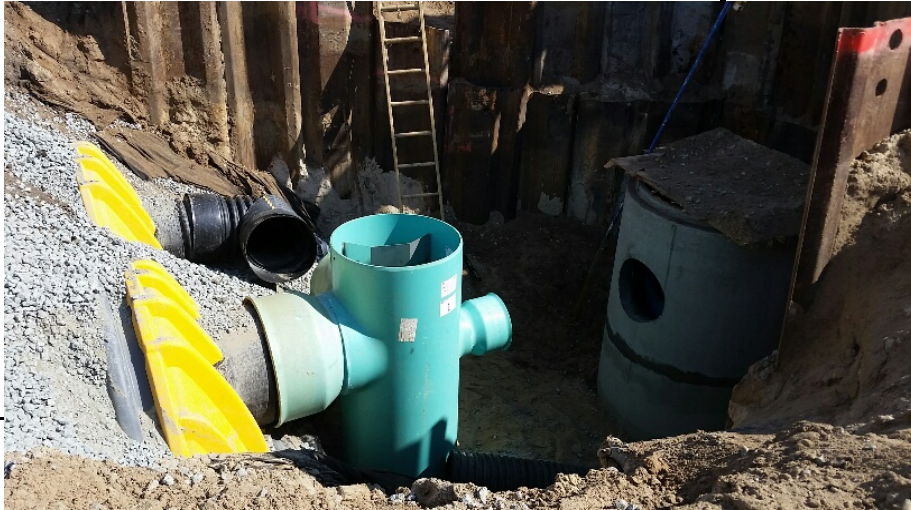
Hydrodynamic Separator #1, weir, and exposed infiltrator, before backfill
