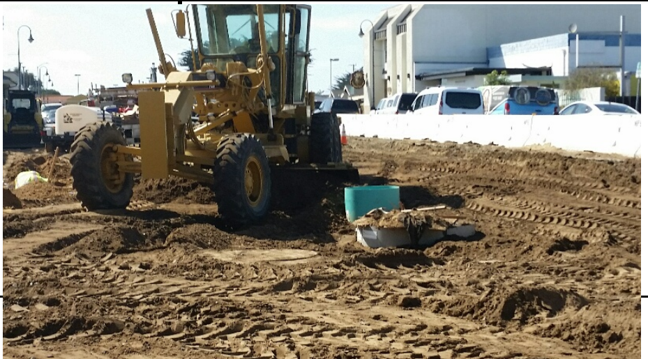
Final backfill and compaction, Hydrodynamic Separator #1
