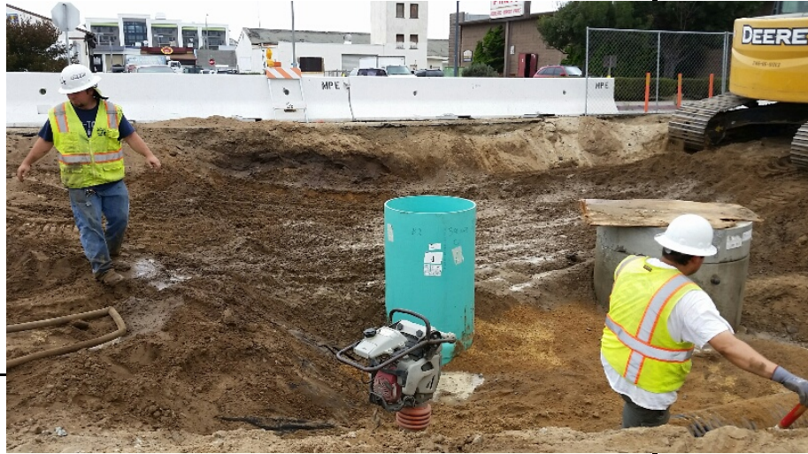
Final backfill and compaction, Hydrodynamic Separator #1
