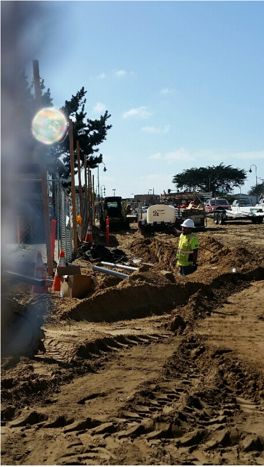
Trench for electrical conduit for streetlights west of Hillsdale Street.
