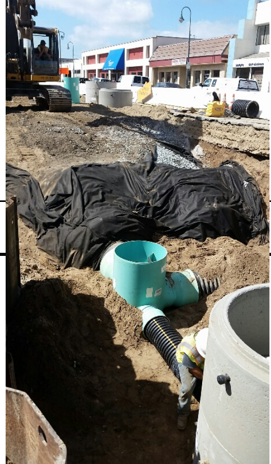
Weir and connecting pipe, HDS #2
