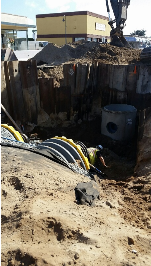
Installation of HDS #2+D12:J39
