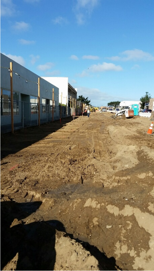
Sidewalk subgrade grading and compaction between Hillsdale and Alhambra Streets
