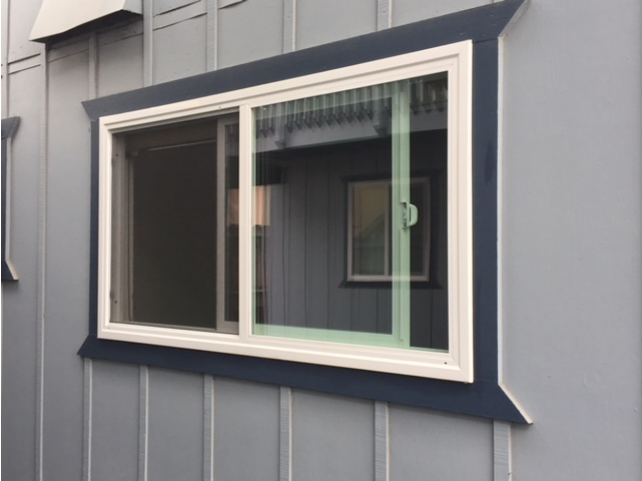
CDBG Funds used to replace windows at Genesis House/Community Human Services
