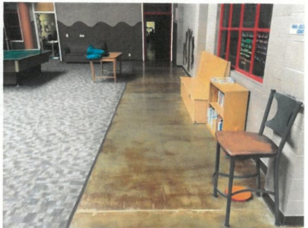
Activity Floor Walk Way start to finish from quarry tile to custom colored stained concrete.
