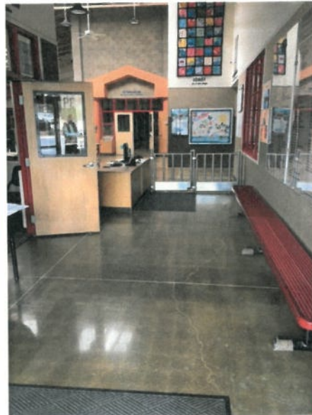
Front Entrance start to finish from quarry tile to custom colored stained concrete.
