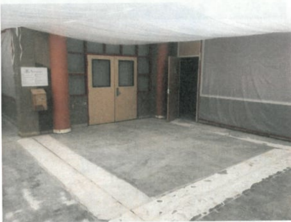
Activity Floor start to finish from quarry tile to custom colored stained concrete.
