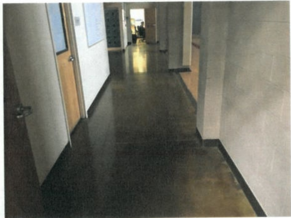
Gym Hallway start to finish from quarry tile to custom colored stained concrete.
