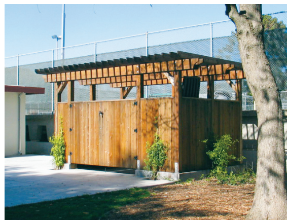
Screened trash enclosure.
