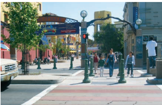
Raised median and bollards at pedestrian crossing increases pedestrian safety.
