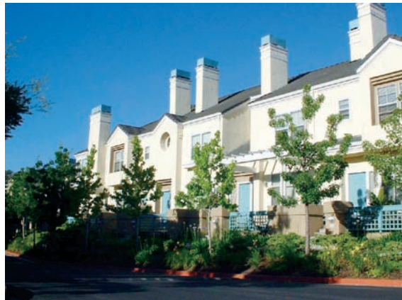
Façades define individual units and residences.
