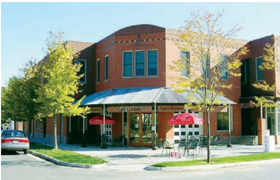
Building set back at corner to provide space for outdoor dining.
