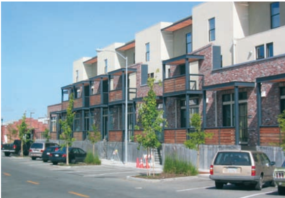
Entries and porches separating mass of multi-story buildings.
