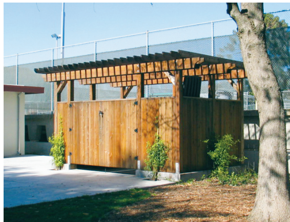
Screened trash enclosure.
