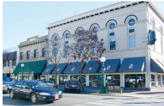
Awnings shaping pedestrian space at the base of buildings.
