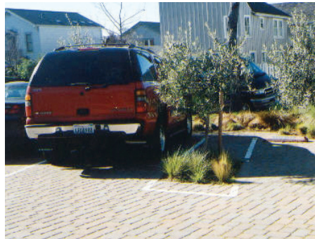
High-quality, permeable brick paving.
