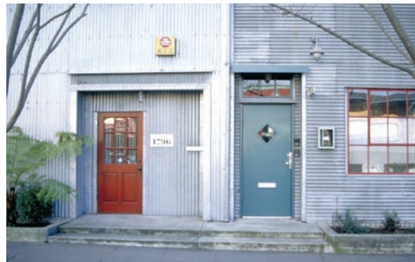
Corrugated metal used in live-work units.
