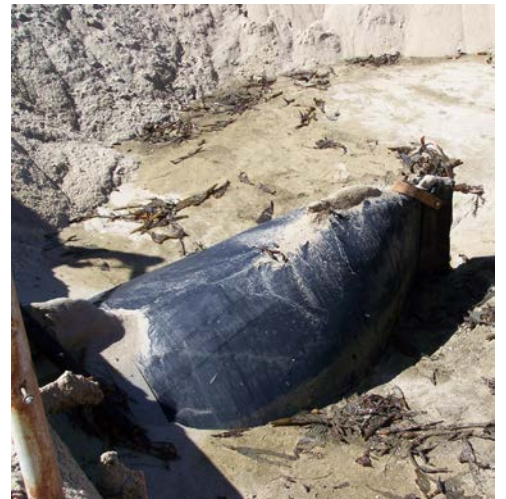
Lower Tideflex check valve blocked by sand
