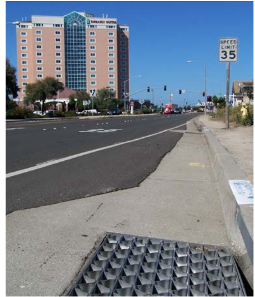
Drainage inlets east side of Canyon Del Rey Blvd.
