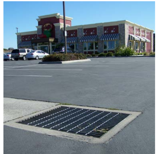
Drainage inlet in parking lot that contributes flow to the deficient pipe
