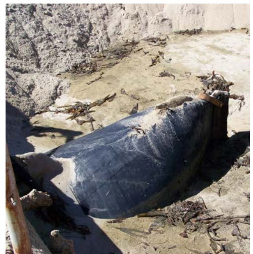
Lower Tideflex check valve blocked by sand
